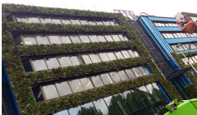
▲ Greenhouse Antwerp - Placement green façade
