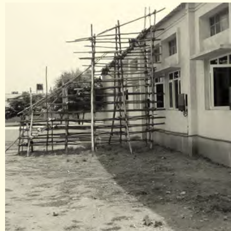
SOLAR PLANT CONSTRUCTION - INDIAN STYLE Via a bamboo staircase, modules and inverters for the PV system are transported onto the roof of the factory.
