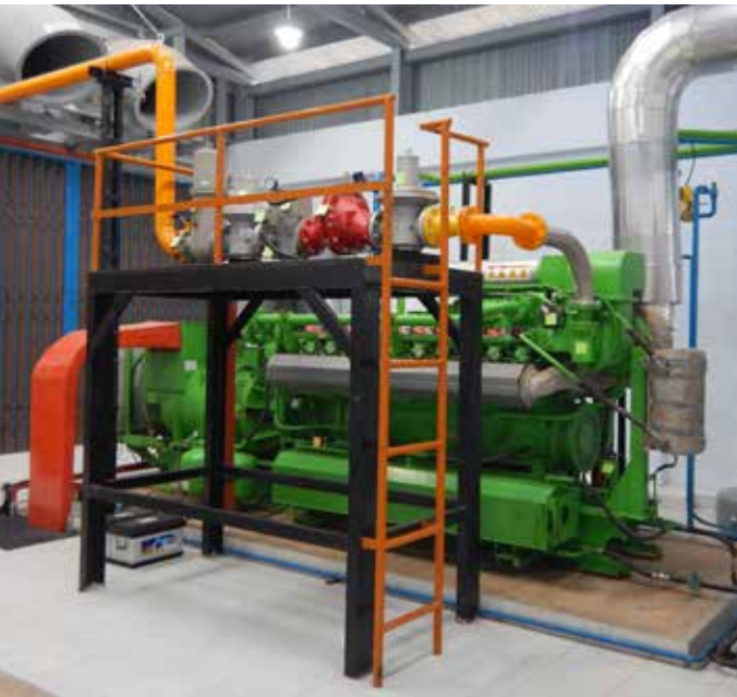
Biogas engine in Mukomuko
