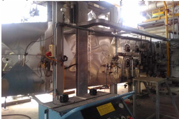
Figure 1 - Channelling of emitted fumes into the steam recovery boiler of the co-generation system
