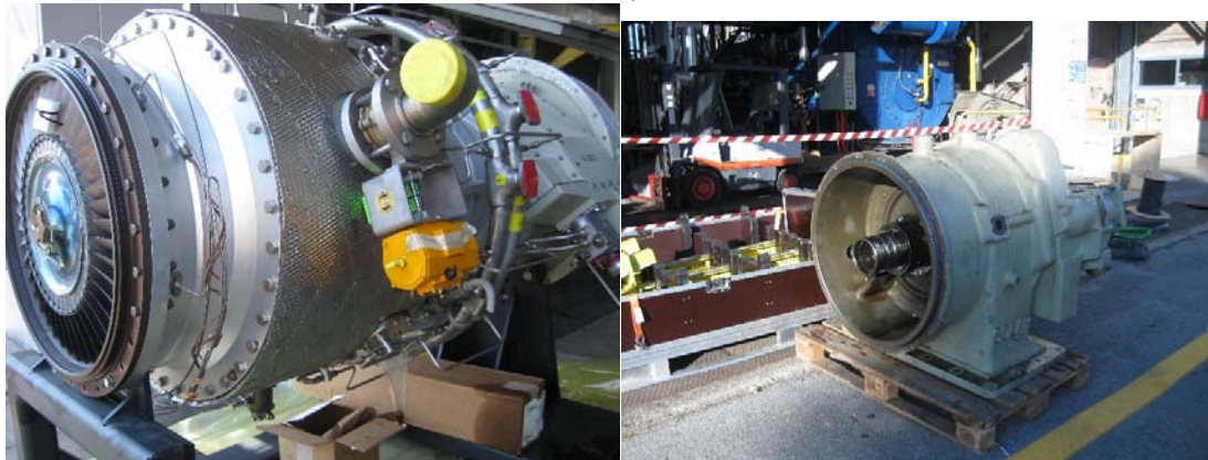
Figure 2 - The gas turbine during its replacement (left); the dismantled reduction gearbox during installation (right) (August 2016)
