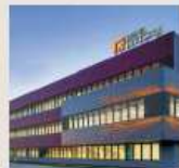
PRIMA INDUSTRIE HEADQUARTERS AND TECH CENTER Collegno (TO) - Italy
