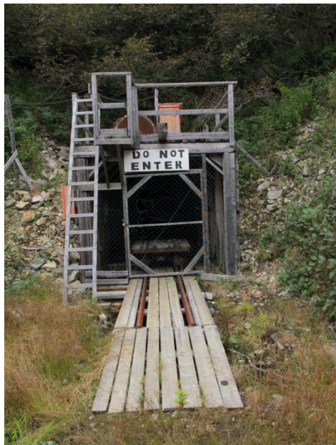
Adit entrance showing ventilation fan
