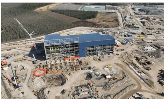
Site Layout - Looking East (CNW Group/Foran Mining Corporation)
