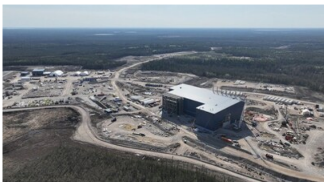
Site Layout – Looking West (CNW Group/Foran Mining Corporation)
