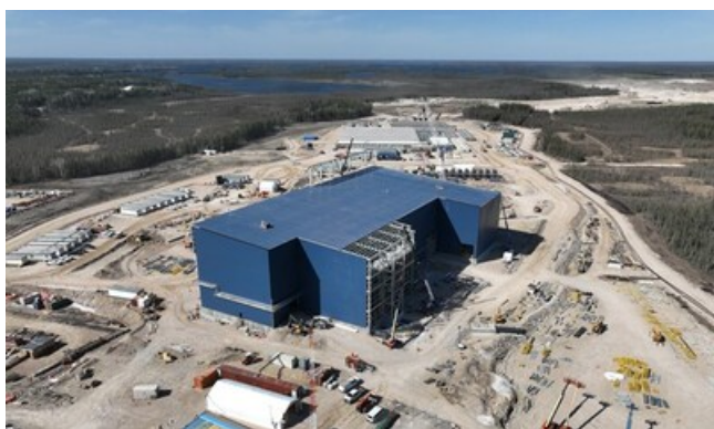
Site Layout - Looking North (CNW Group/Foran Mining Corporation)
