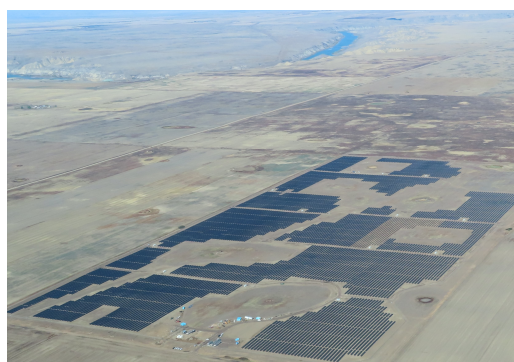
Empress solar project, Empress, Alberta, Canada
