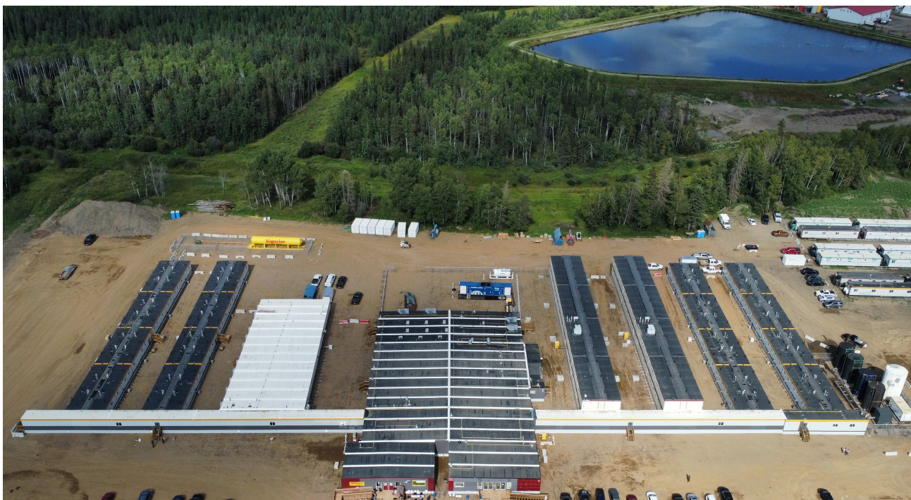
Fire Relief Camp, High Level, Alberta, Canada
