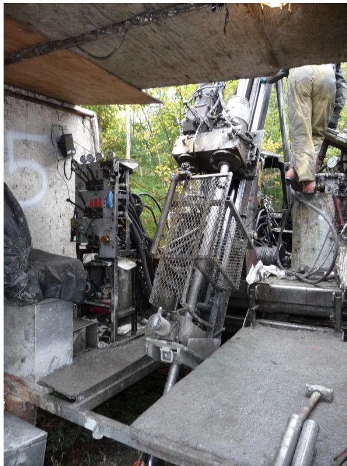
Hole AL-10-08 drill setup
