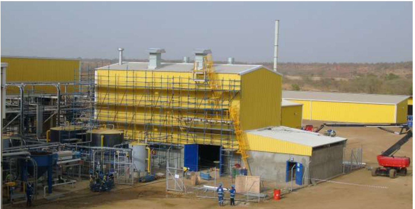
Cladding of Gold Room Nearly Complete
