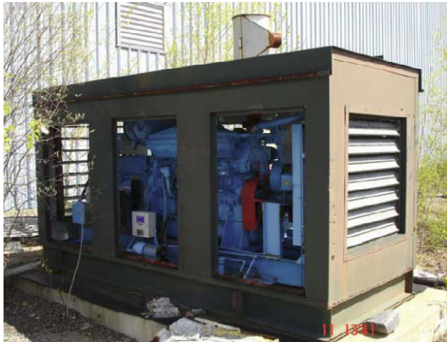
Figure 4-4. Standby Generator
