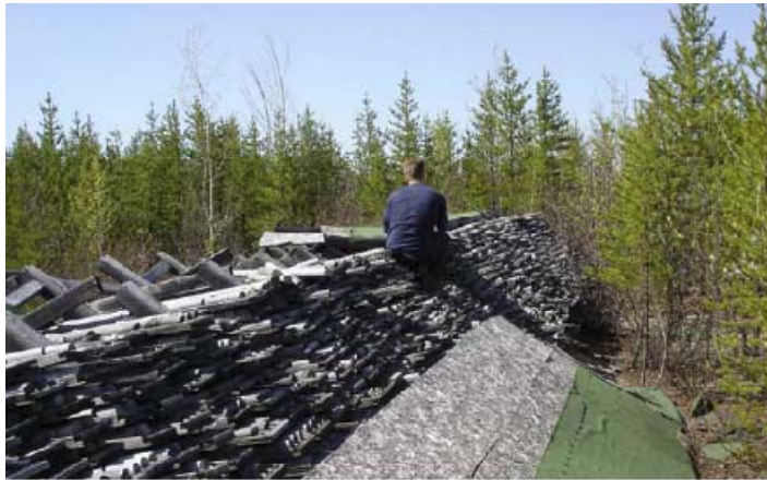
Figure 4-6. Collapsed Core Racks.
