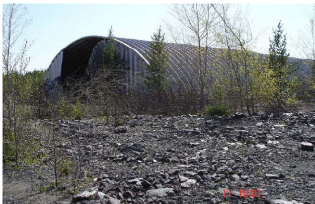
Figure 4-5. Cover over Portal.
