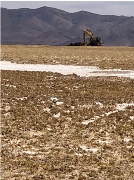
Fig 2 shows the cat 320 trenching in the distance across the salt pan
