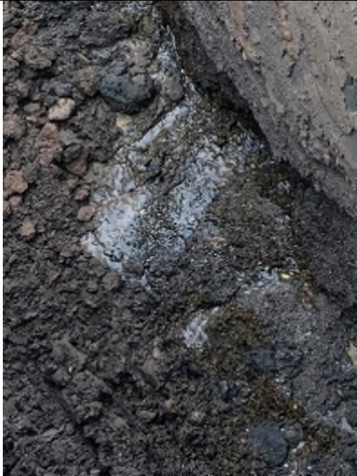
Fig3 shows the transition from the green gray clay possibly montmorillite with black sands/shales/agreggates starting to show through with water seeping immediately
