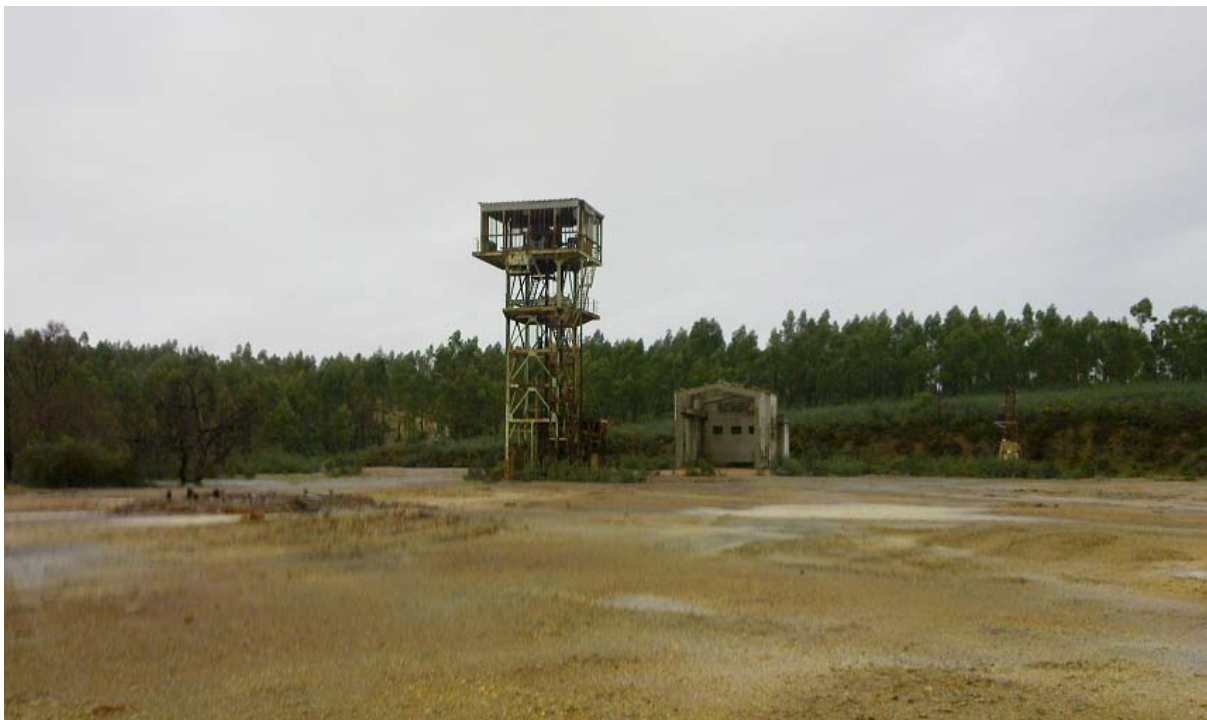
Figure 3 Lomero-Poyatos mine shaft
