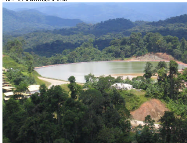
Figure 13 View of Tailings Pond
