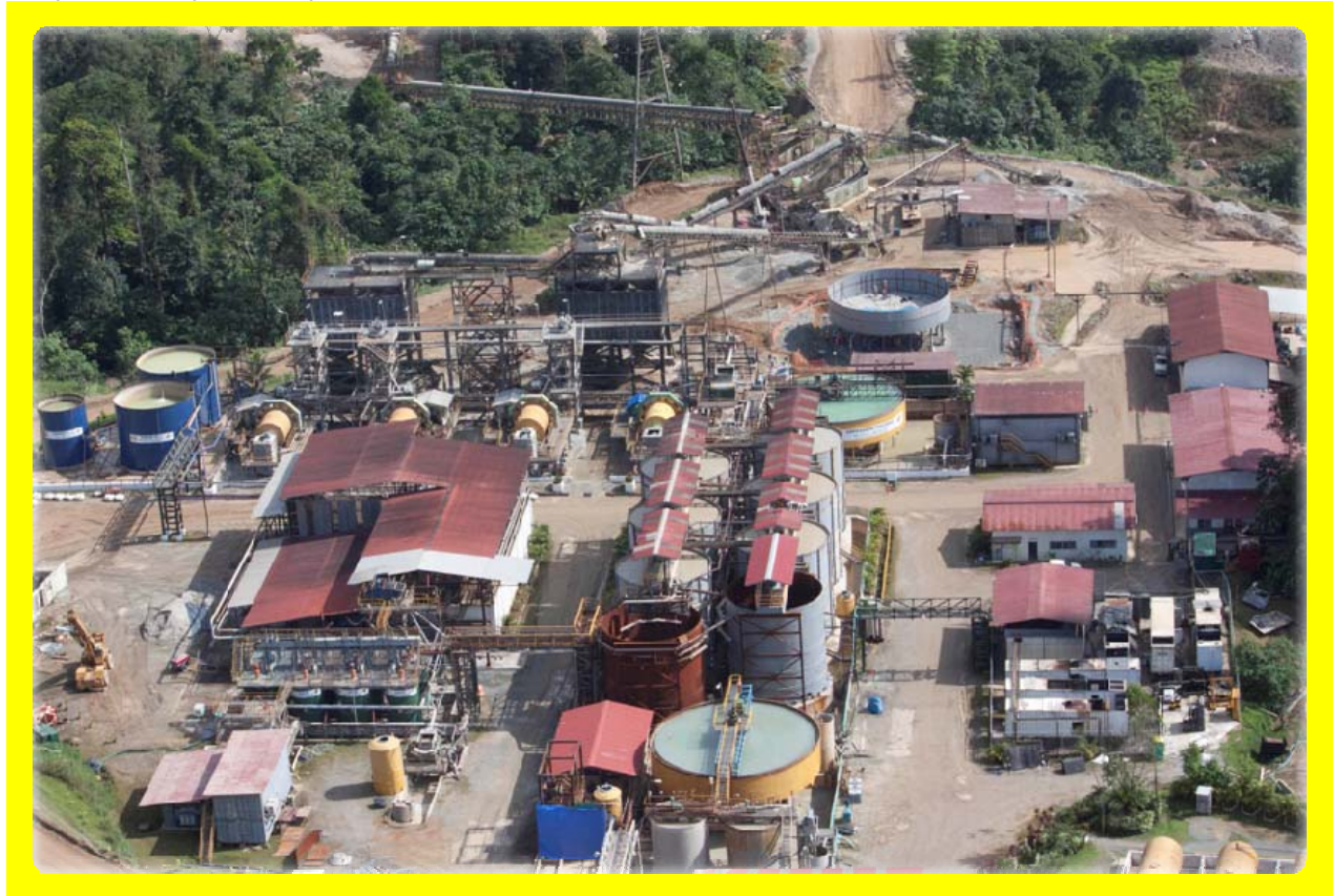
Figure 6 Molejon Gold Project – Molejon Gold Plant
