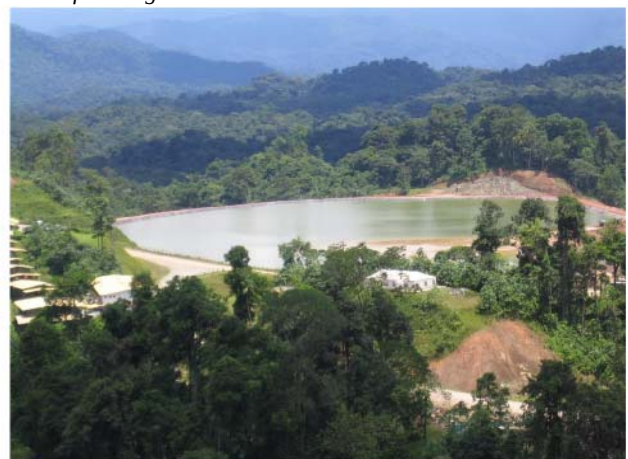
Figure 13 View of Tailings Pond
