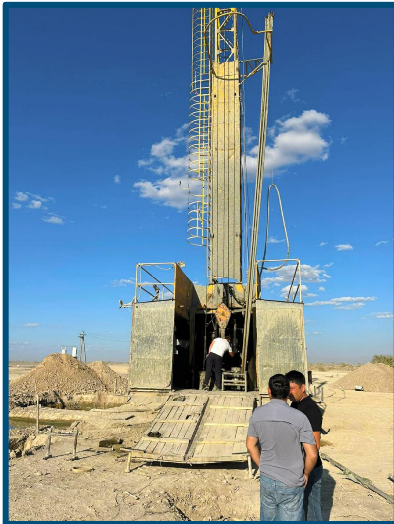
Setting up Drill Rig at Chu-Sarysu, Kazakhstan
