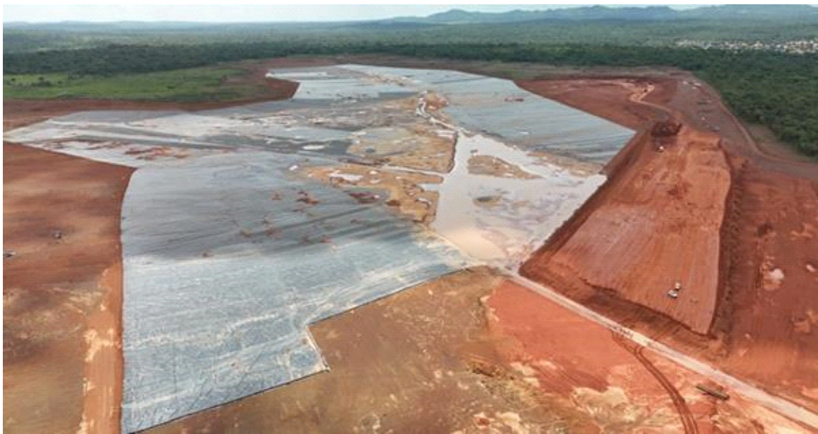
Figure 4: Tailings storage facility showing the extent of lining and main embankment construction (11 July 2025).
