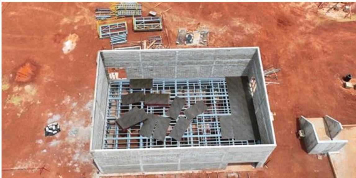
Figure 9: Aerial view of the HV Switchroom (15 July 2025)
