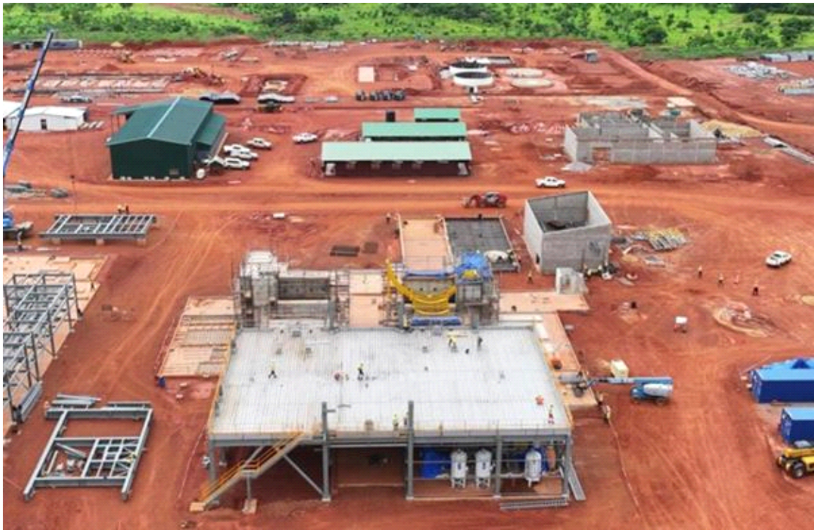
Figure 2: View of Milling building showing erection of steel (15 July 2025)
