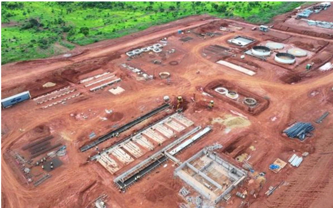
Figure 8: Five out of eight power station generator bases have been poured (7 Jun 2025)
