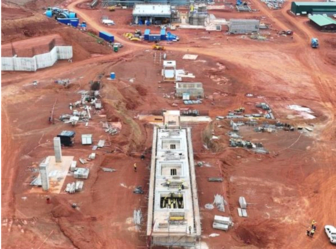
Figure 7: View of reclaim chamber (15 July 2025)
