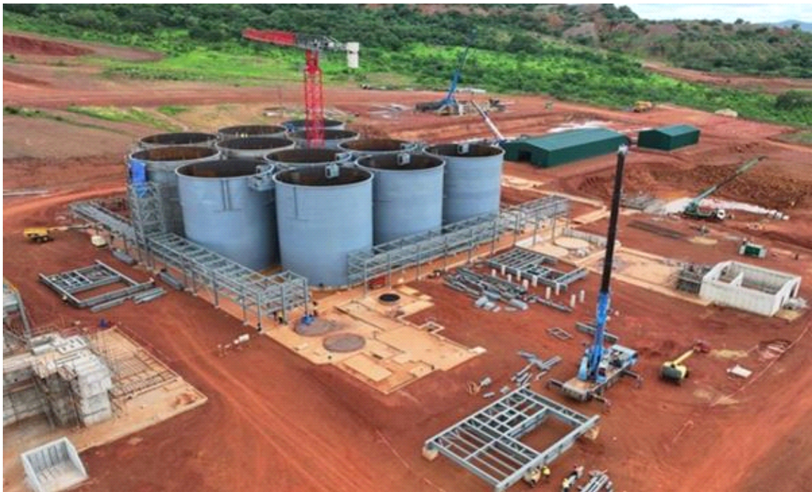
Figure 3: View of CIL with pipe rack and top of CIL tank steel erection (15 July 2025)
