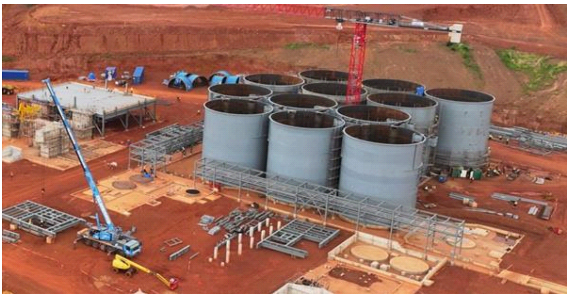
Figure 5: View of CIL tanks all at full height (15 July 2025)
