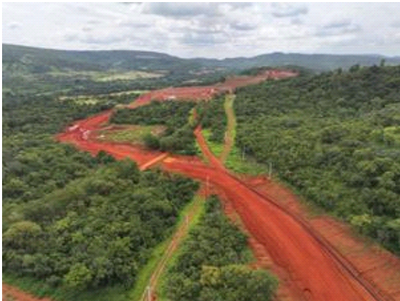
Figure 13: Overland piping installation (12 October 2025)
