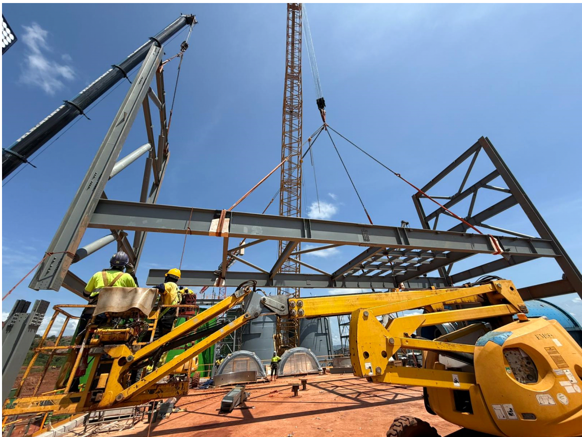
Figure 3: Mill classification tower steelwork lift (13 October 2025)
