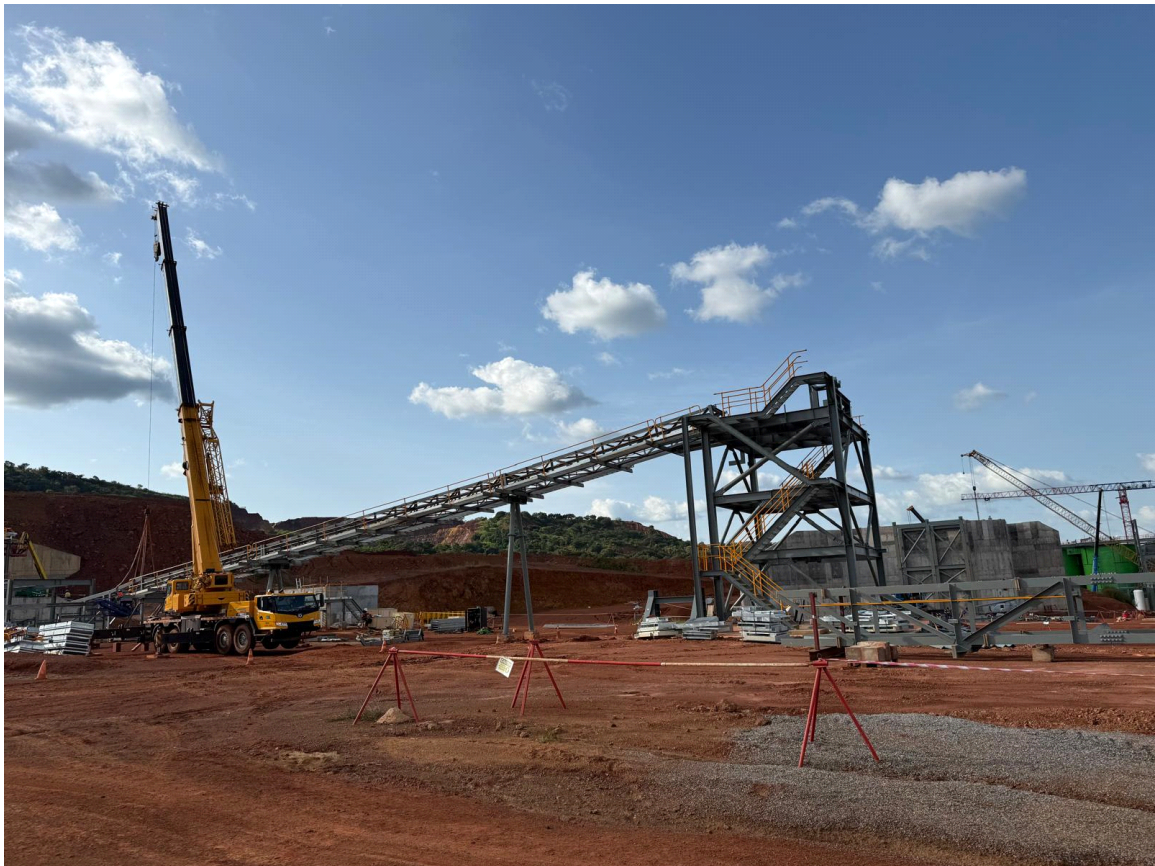
Figure 5: Stockpile feed conveyor truss modules erection (13 October 2025)
