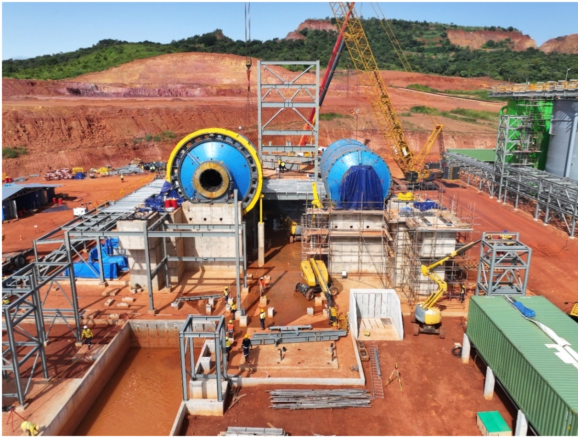
Figure 2: View of milling building showing mill suspended slab complete and mill installation (12 October 2025)
