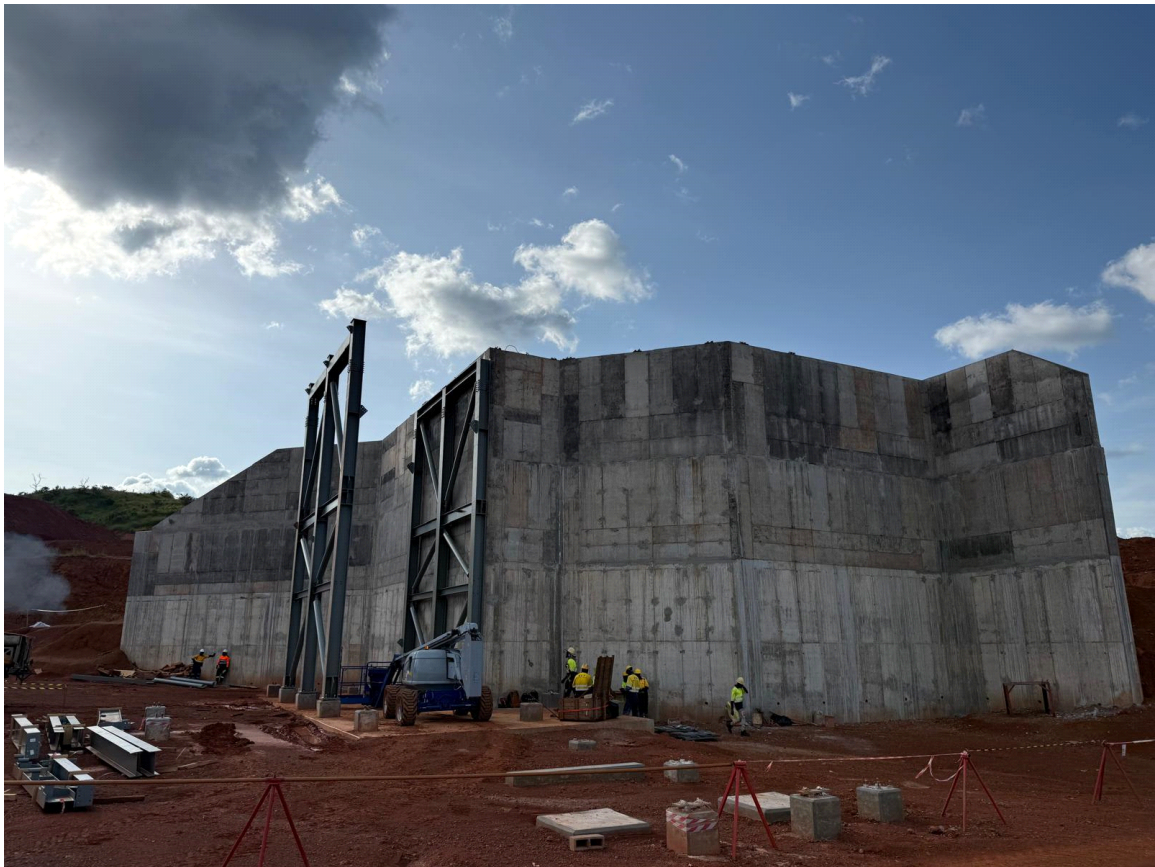
Figure 8: Oxide crushing steel erection progress (13 October 2025)
