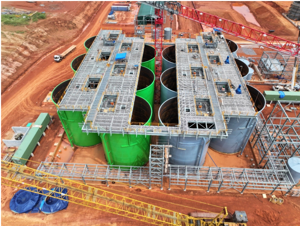
Figure 6: View of CIL with pipe rack and top of CIL tank steel erection (12 October 2025)
