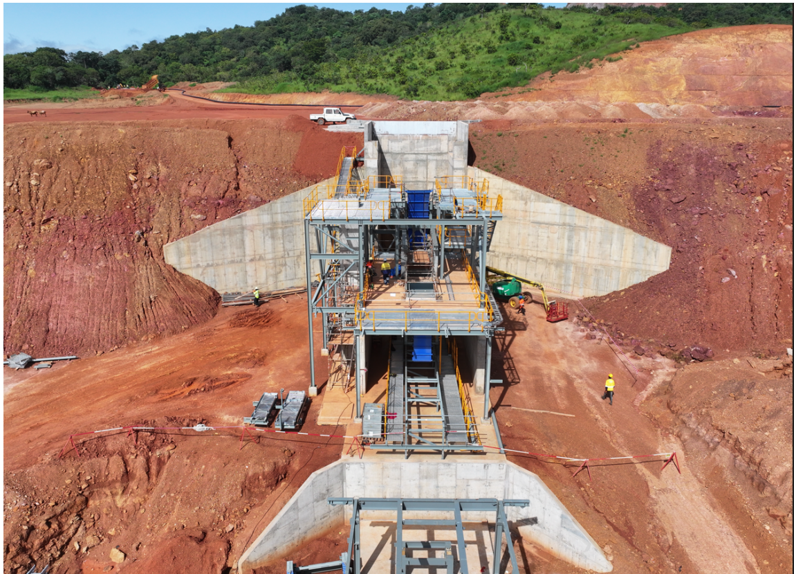
Figure 7: Primary crusher steel erection progress (11 October 2025)
