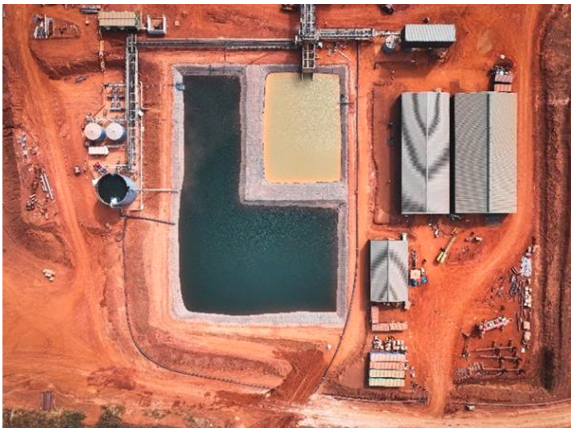
Figure 8: Water Treatment Facility
