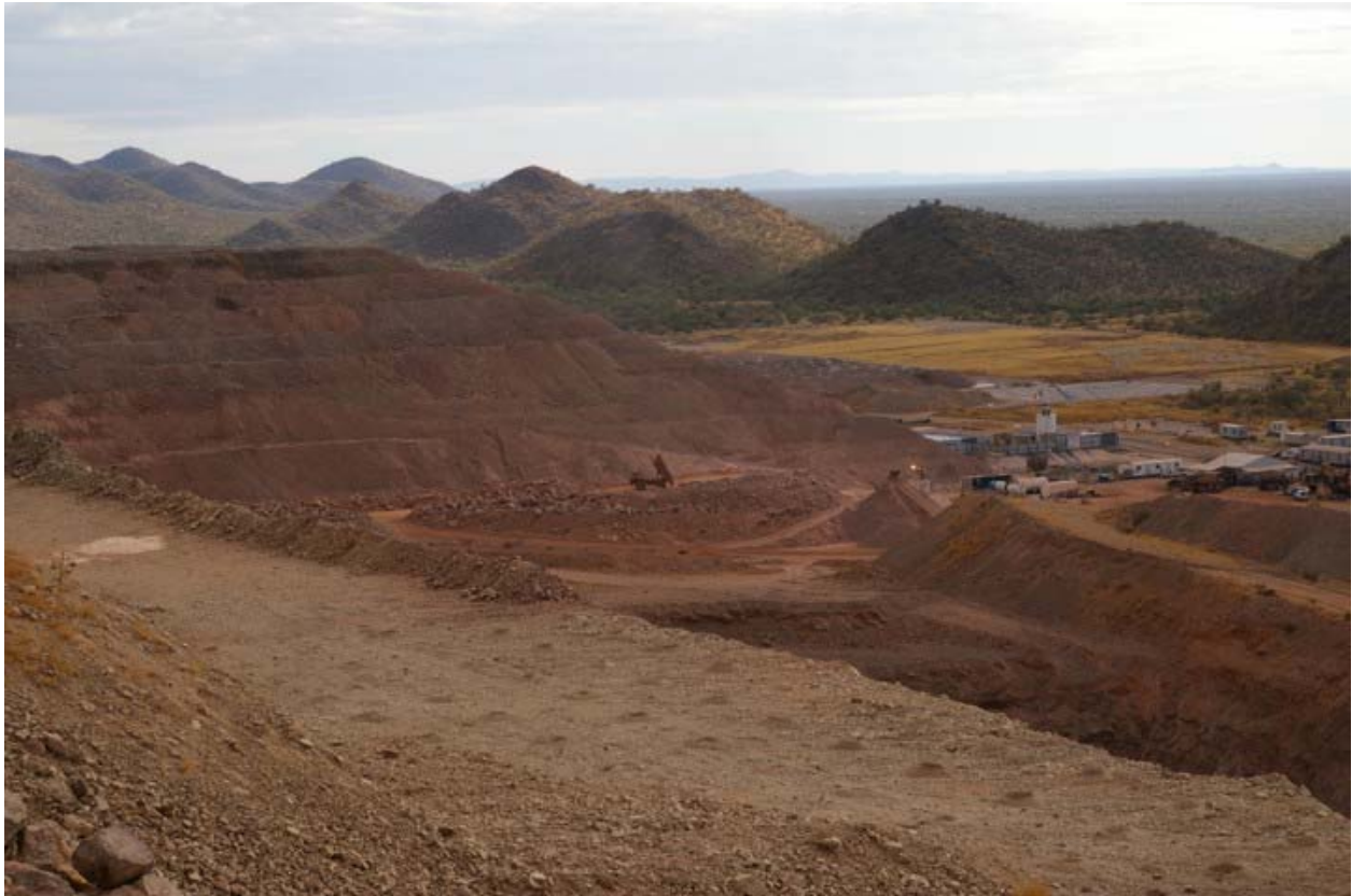
Figure 5-2 Photograph showing the heap leach pads (primary pad on the left and secondary pad behind in the centre) with crushing facility to the right of the toe of the primary leach pad. View is looking to the south east from just north of the Harris pit.
