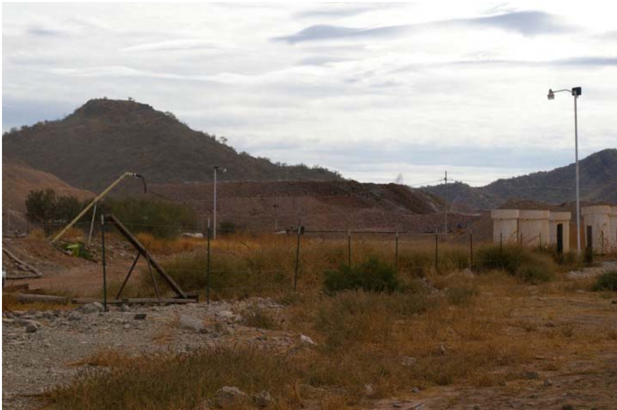
Figure 16-3 Photograph showing the secondary heap leach pad with cyanide sprayers on. Three lifts were completed by the end of January 2009.
