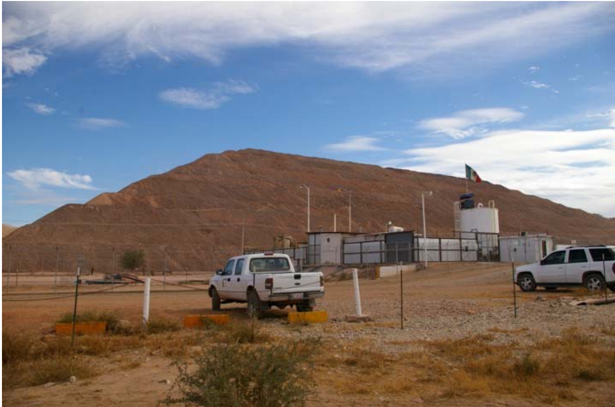
Figure 16-2 Photograph showing the primary heap leach pad behind the processing plant. A collection pond is located in the fenced area in front of the truck on the left side of the photo.
