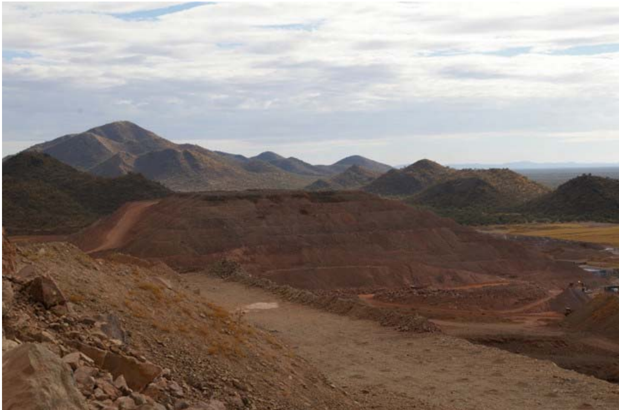
Figure 16-1 Photograph showing the primary heap leach pad (completed) in the foreground. The secondary pad is in the background with cyanide sprayers on.
