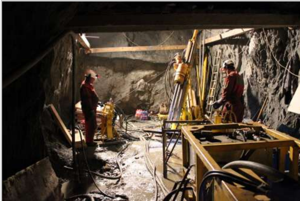
Figure 10-3: November 2012 Underground Drilling (Level 6)
