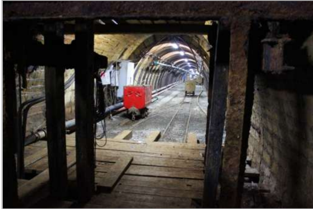
Figure 9-1: Level 6 after Rehabilitation and Pumping
