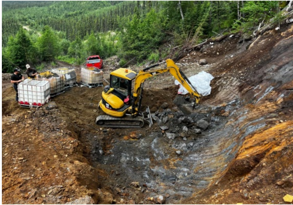
Figure 2: Low-cost surface excavation of outcropping graphite at the Berkwood Project bulk sample site on Zone 6.
