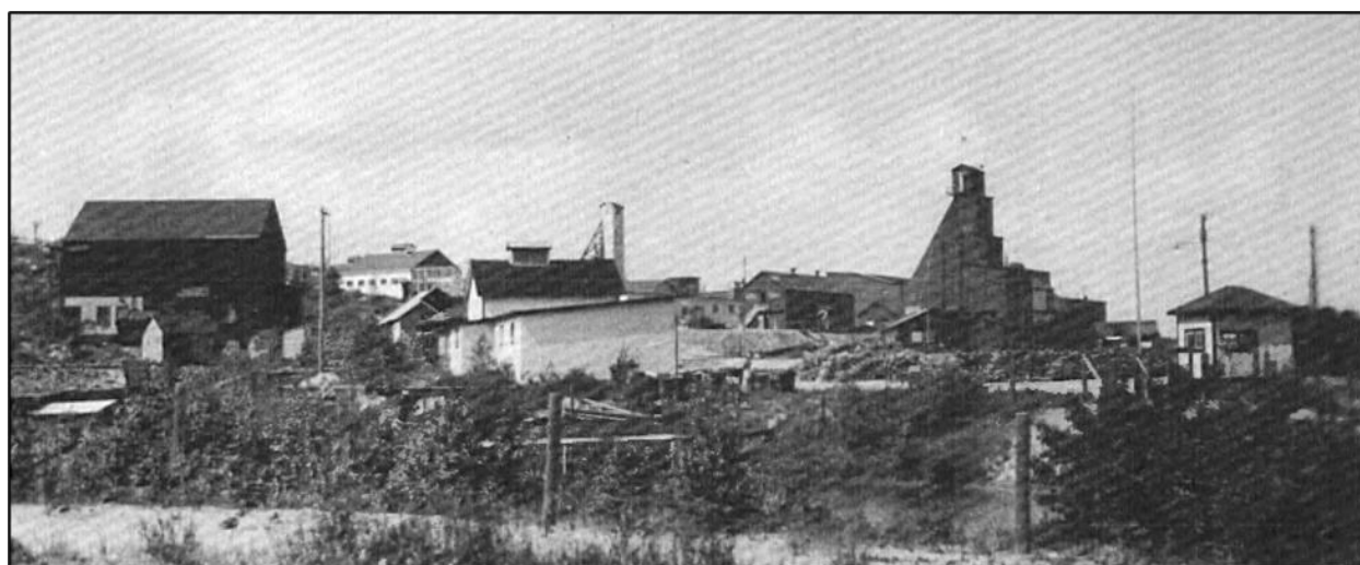
Figure 6–2: Processing Infrastructure of Normétal Mine
