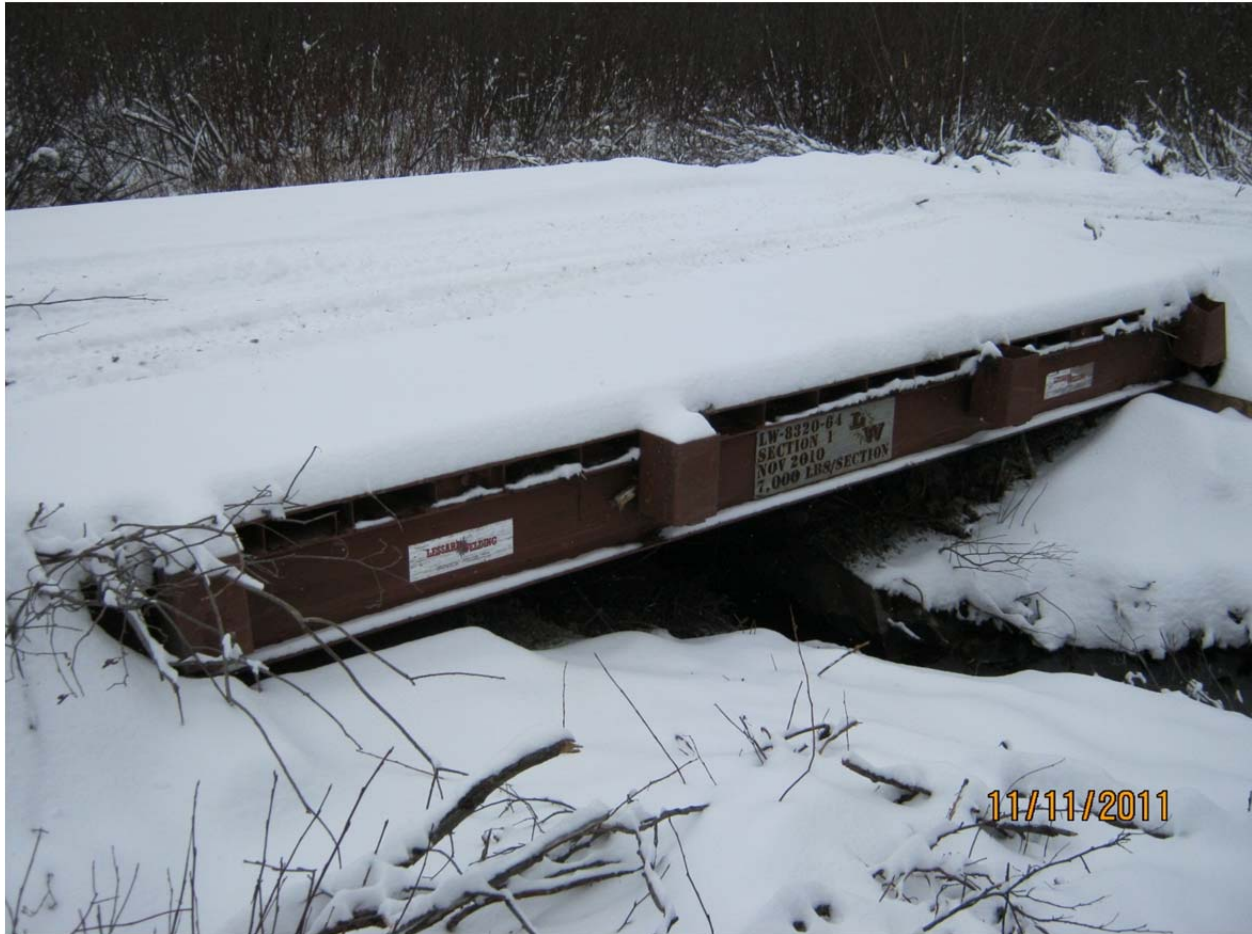
Figure 4-6 Photo of temporary bridge on the road close to Line 60 property.
