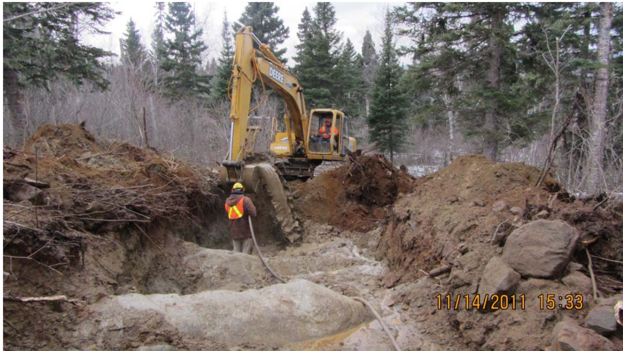
Figure 9-6 Trenching in progress at channel L60-11-C06.
