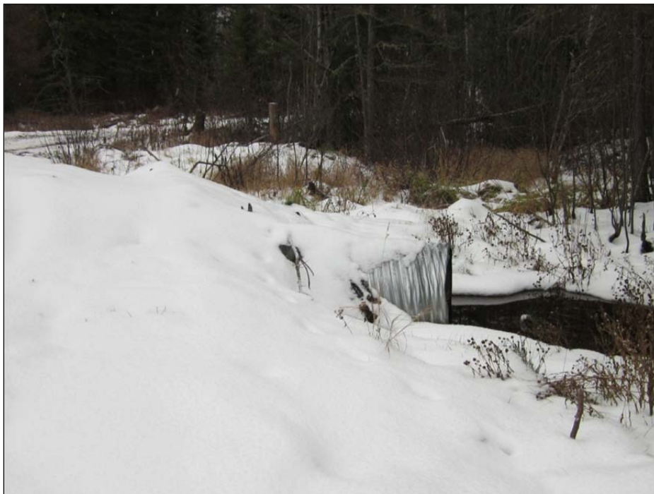
Figure 12-4 Metal culvert on Nama Creek Road
