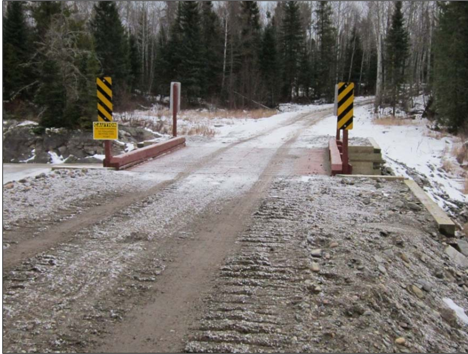
Figure 12-3 : Permanent bridge on Nama Creek Road
