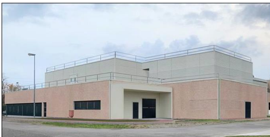
Biotech Rosia Production - Rosia Plant (Siena)
