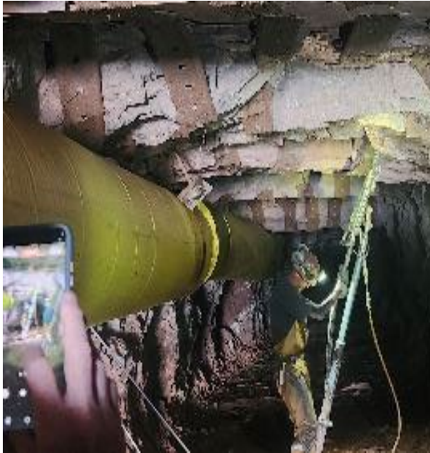
View of rock bolting roof in the decline
