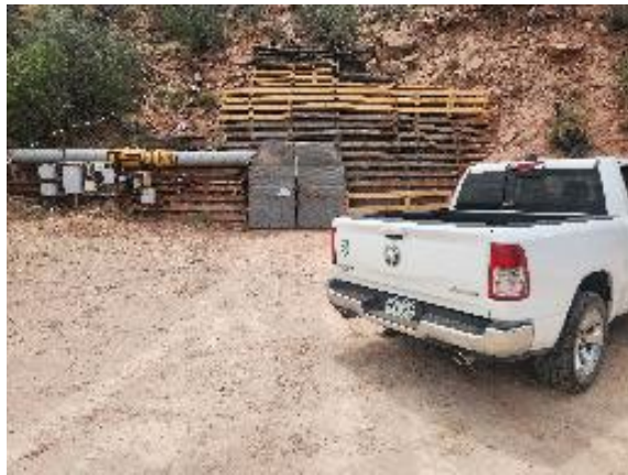
View of JD8 mine portal with ventilation system visible
