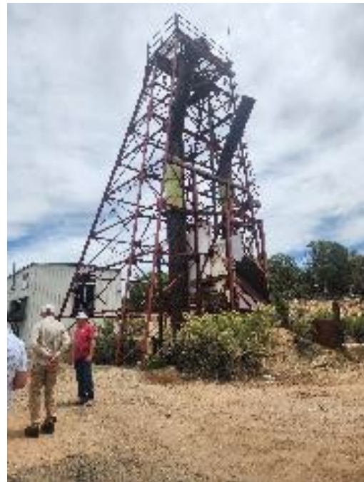
View of JD5 shaft and hoist building
