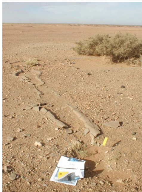
Figure 14.7 Presumed collar location of drillhole I53 (centre foreground) showing remains of concreted drainage channel and sump (in front of bushes)
