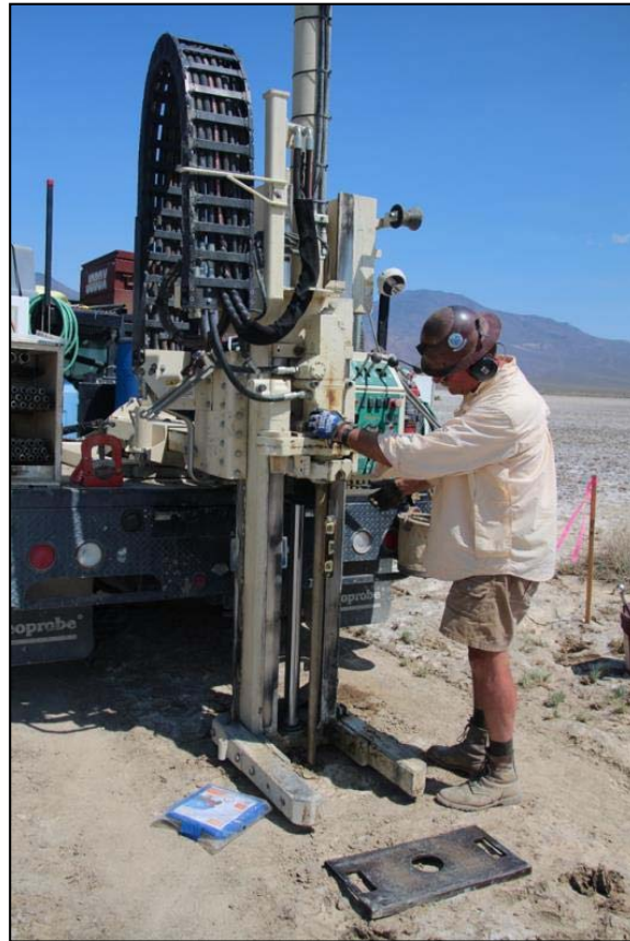
Figure 10-1. The Geoprobe in operation drilling a hole at Teels Marsh.
