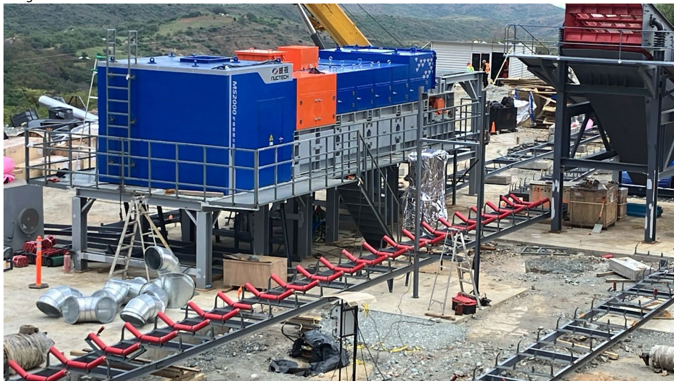
Image 2: Ore Sorter Install
