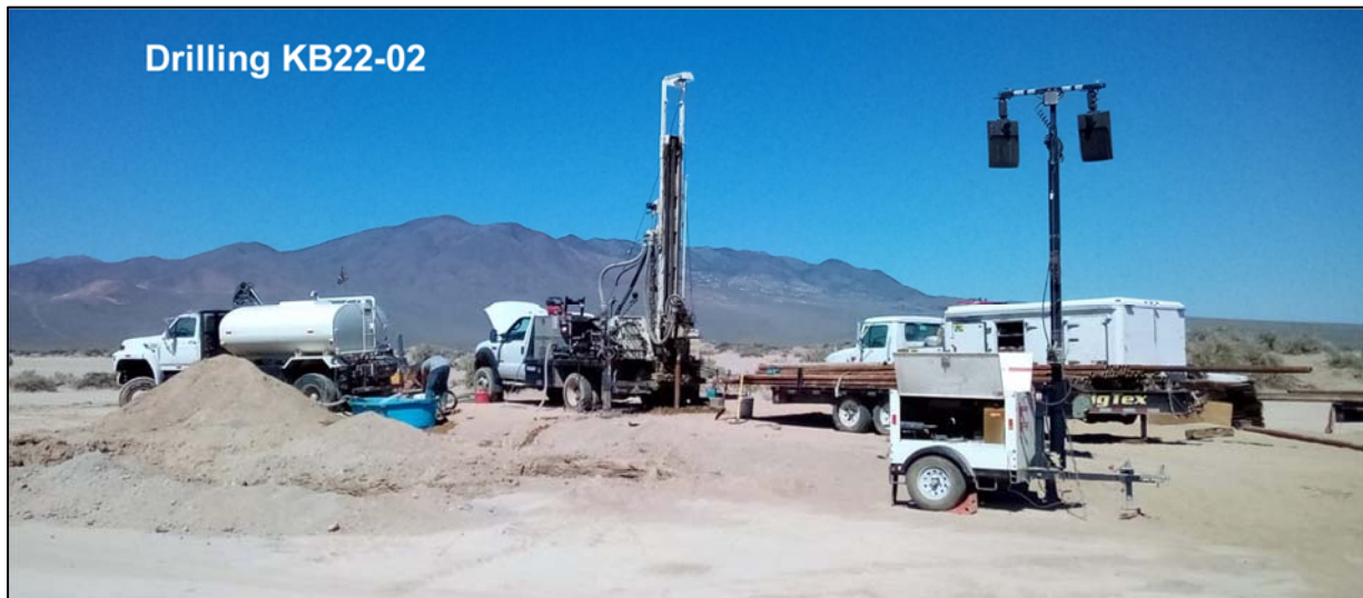
Drilling KB22-02 Completed. Down Hole Packer Water Testing In Progress
