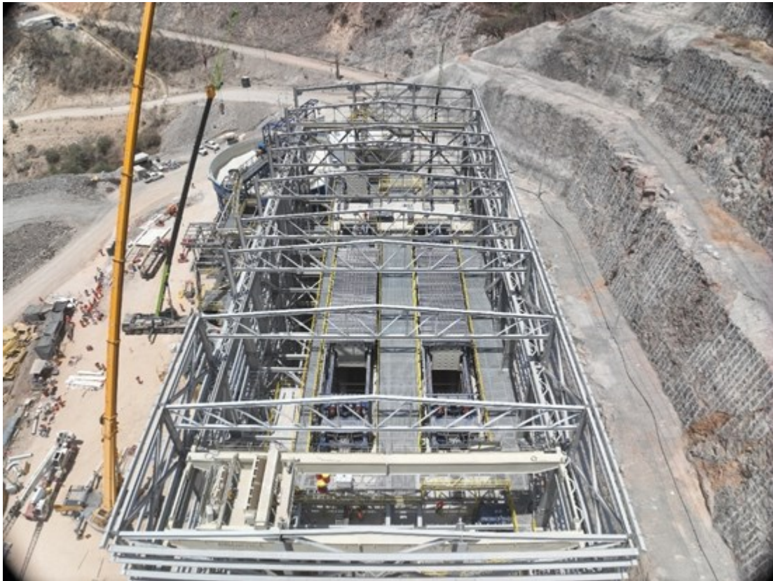
Figure 3: Paste plant filter installation.
