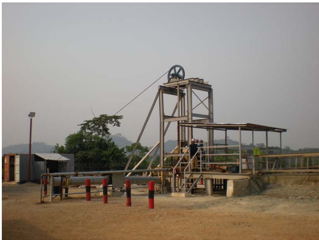
Photo 12 Bardu Shaft, Kono
