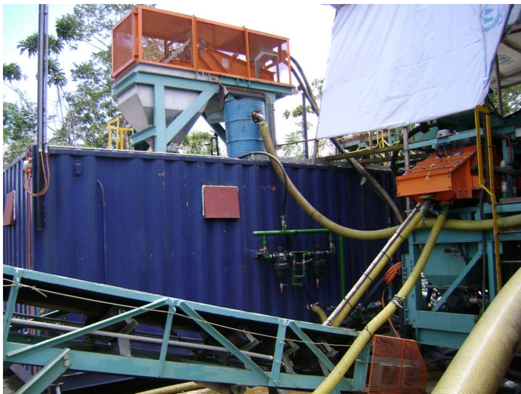
Photo 5 Weasua Plant, X-ray Recovery Unit Showing Direct Feed From DMS
