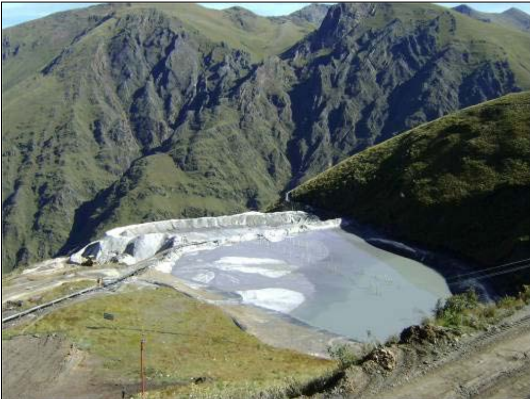
Photo 20: Tailings pond after construction
