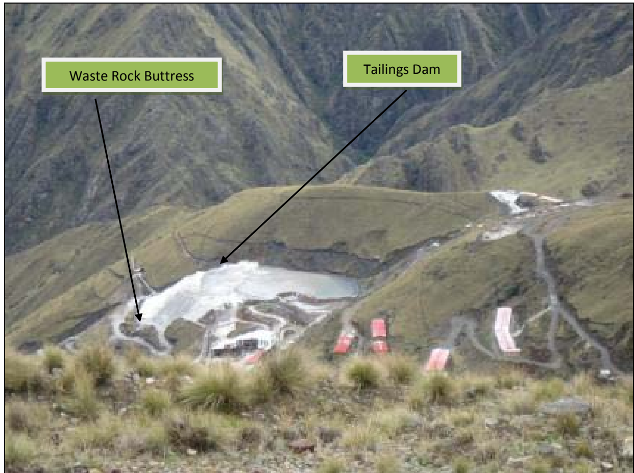
Photo 18: View above Huaura Mill looking east at existing tailing storage facility.
