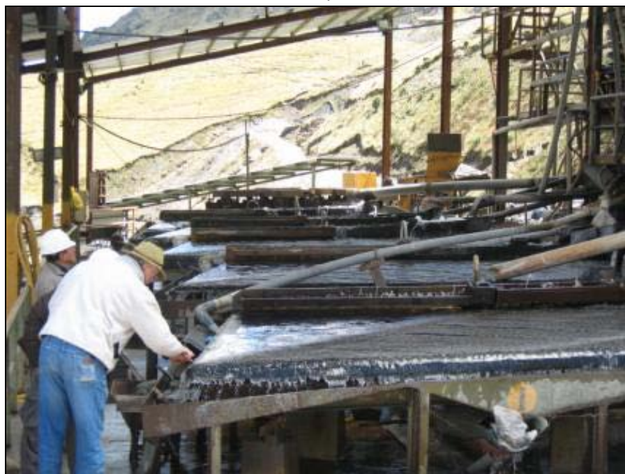
Photo 13: Vibratory tables (bank A)
