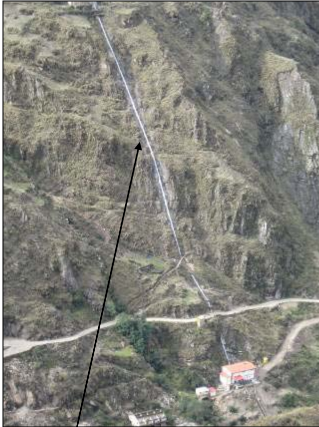
Photo 6: Penstock feed to hydroelectric plant.
