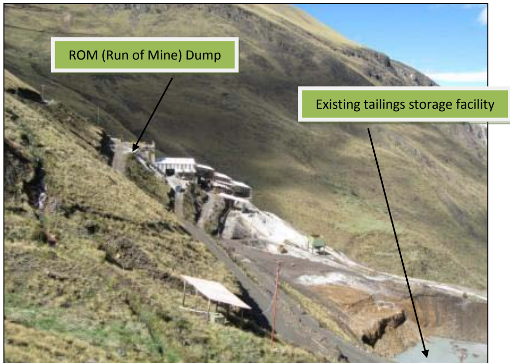
Photo 7: View looking west toward Huaura Mill.
