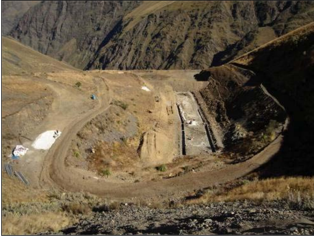
Photo 19: Tailings pond during construction
