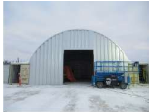
Temporary truck shop
