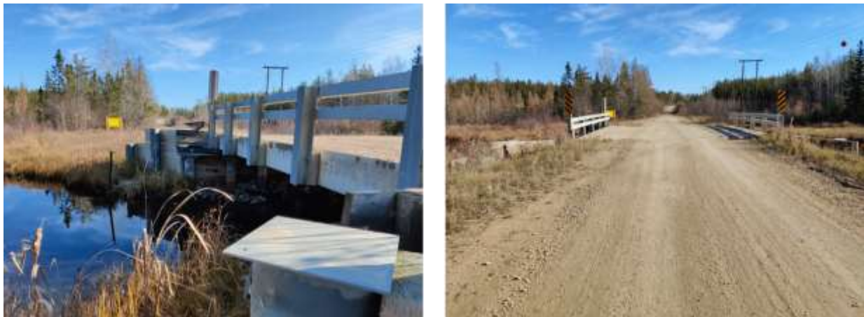
Figure 18-7: Mcllvenna Bay Site Access Road Bridge
