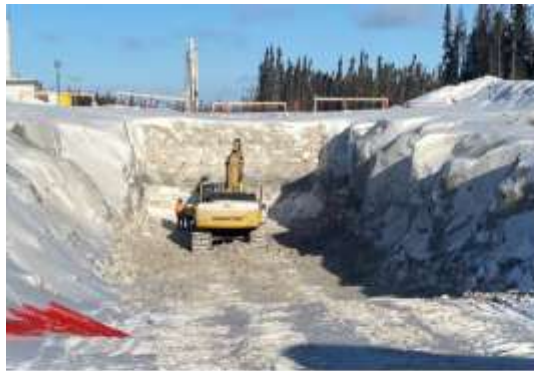
Box cut for portal development
