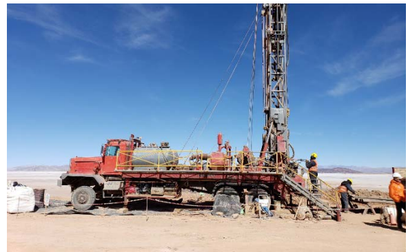
Drill rig onsite at NRG HMN Lithium project.
