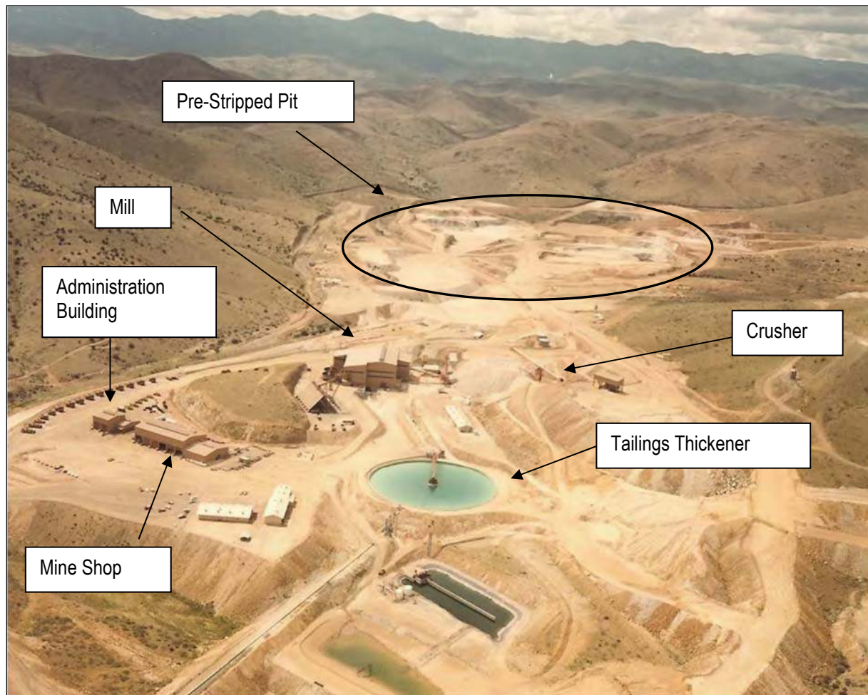
Figure 6-1: Copper Flat Mine in 1982
