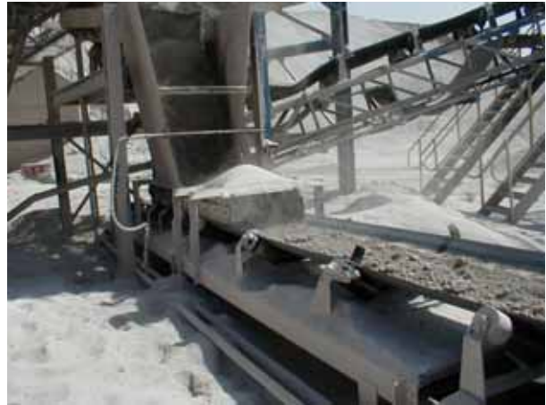
Ore on conveyor from jaw crusher to plant
