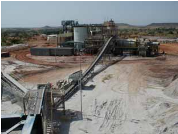
Samira Hill Gold Project CIL Plant
