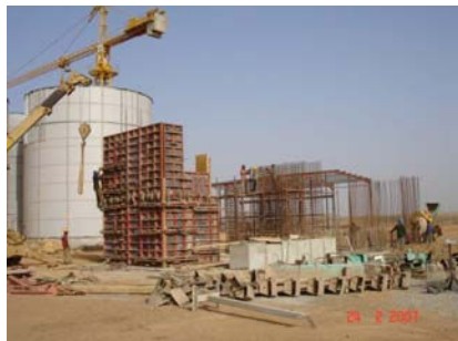
Installation of rebar and forms for ball mill foundation
