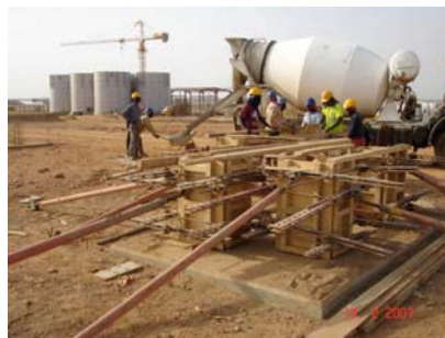
Pouring of conveyor foundations with completed CIL tanks in background
