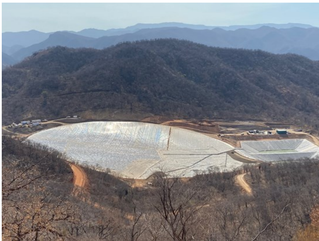
Photo 1 - Santana Heap Leach Pad complete with commencement of stacking earlier this month
