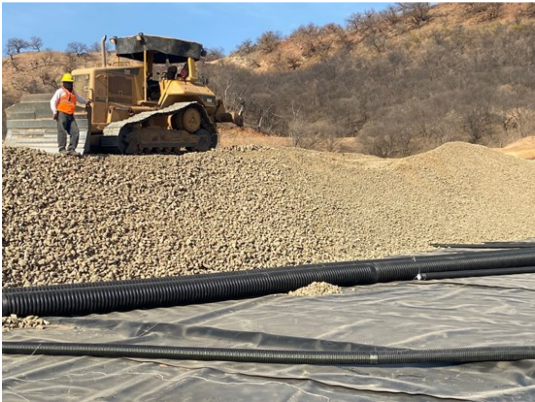
Photo 4 - Heap leach pad loading
