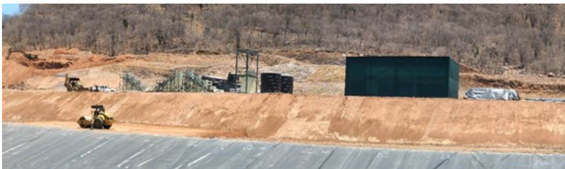
Photo 3 - Gold recovery (carbon) plant completed and awaiting start of commissioning
