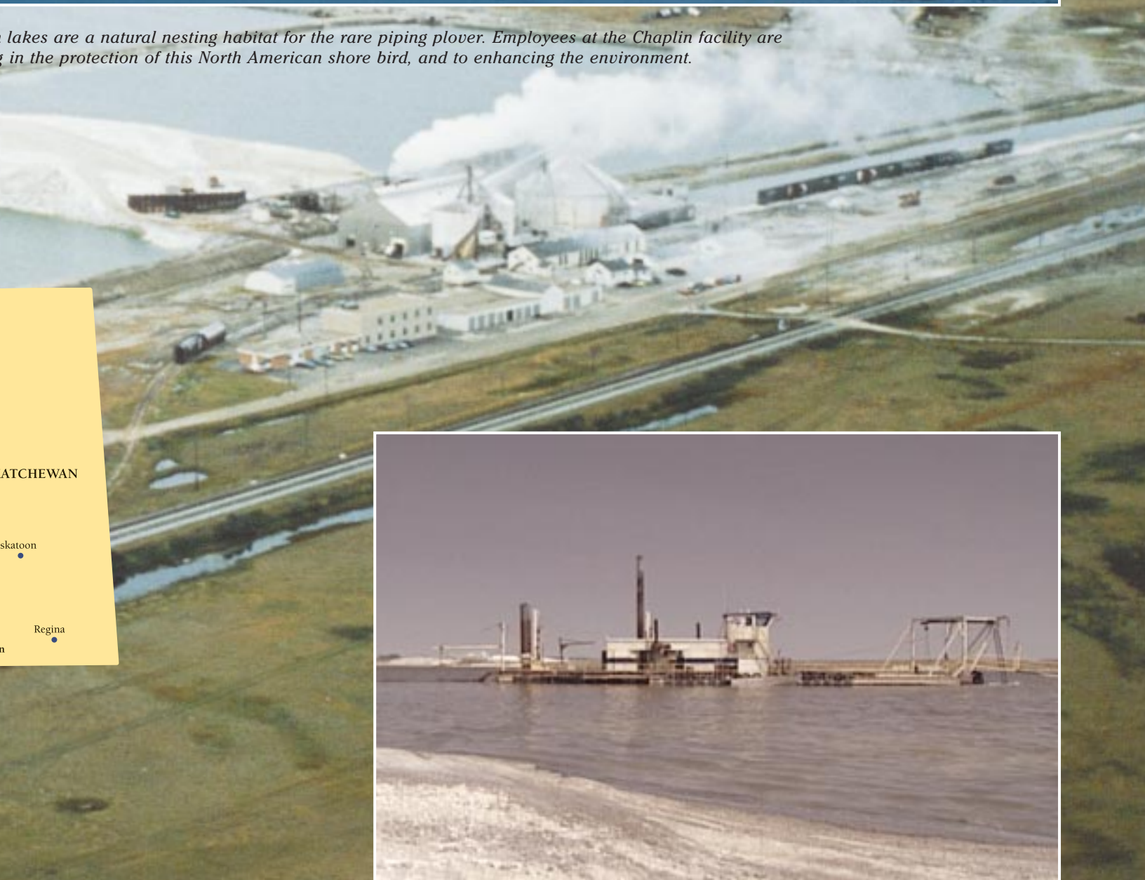
Sodium sulphate at the Ingebrigt facility is recovered from the salt deposit located under a 700 acre lake, by use of a floating dredge, equipped with a cutting head.
