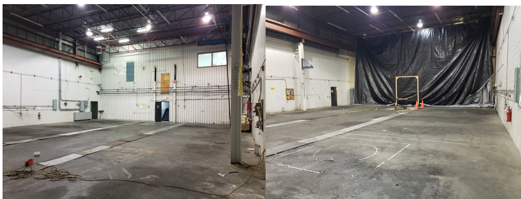
Before Pictures of work area where Gen3 PUREVAP™ pilot plant will be assembled at PyroGenesis plant
