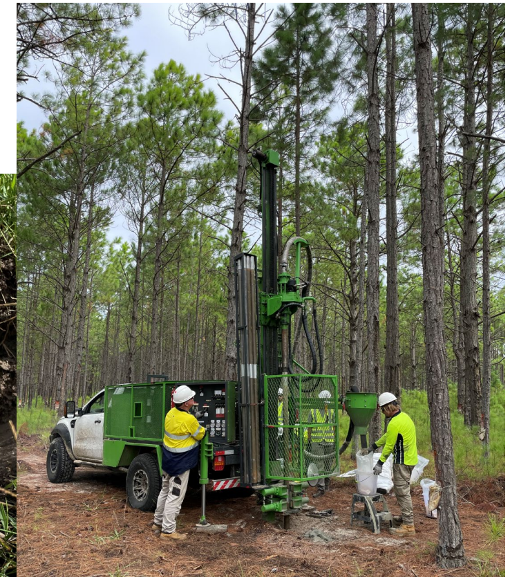
DRILLING ACTIVITIES FEBRUARY 2024
