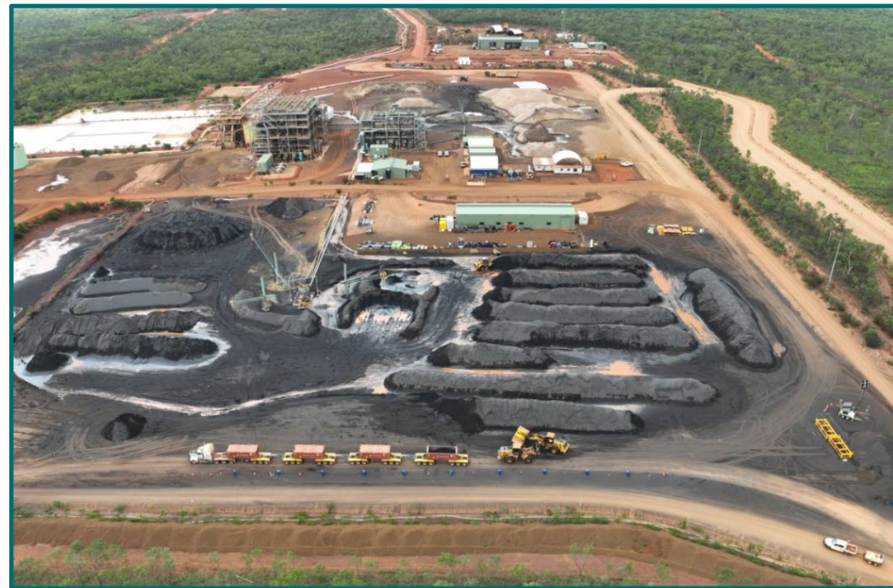
PROCESS PLANT AND PRODUCT STOCKPILES DECEMBER 2024
