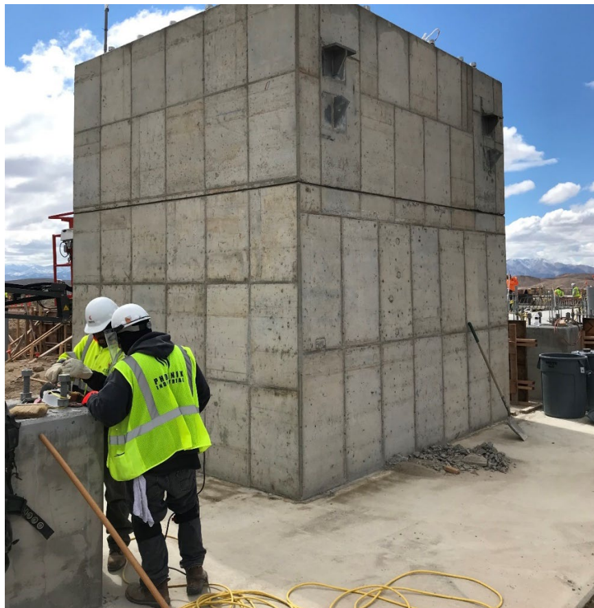
(Completed concrete for the vertical mill)
