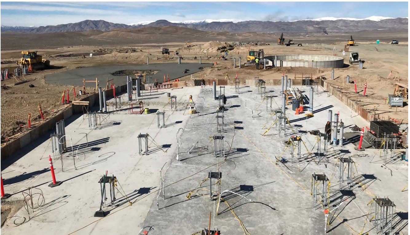
(flotation deck foundation)
