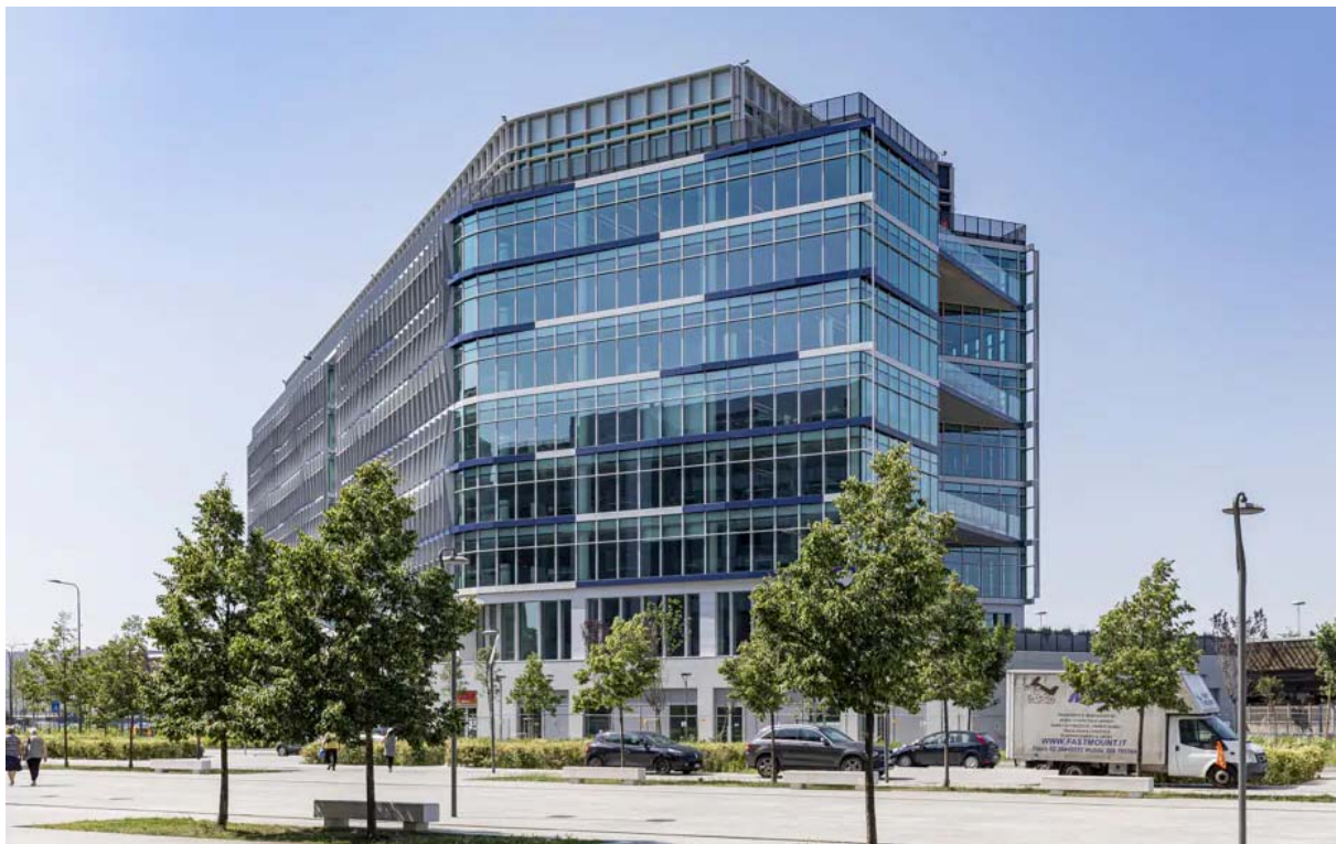
SAIPEM HEAD OFFICE, Spark 1
