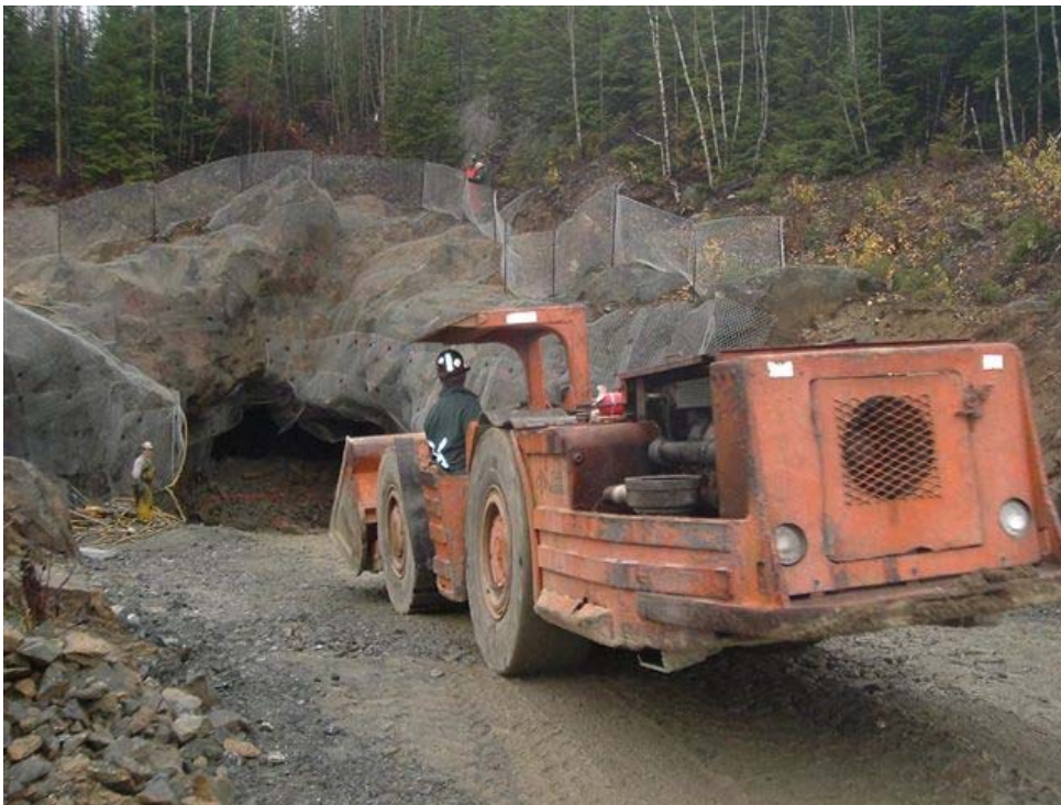
Figure 4: Reopening and securisation of the portal
