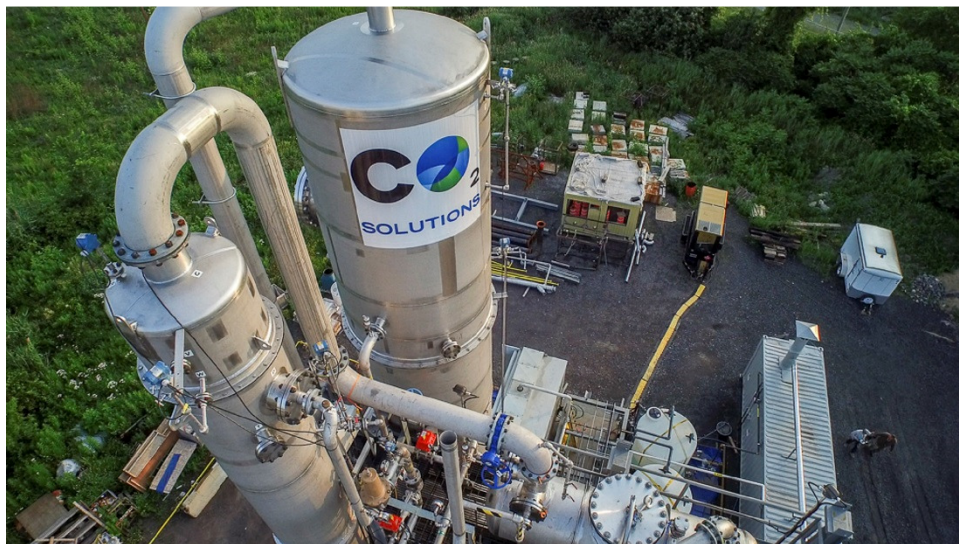
Demonstration Project located at Salaberry-de-Valleyfield, Quebec
