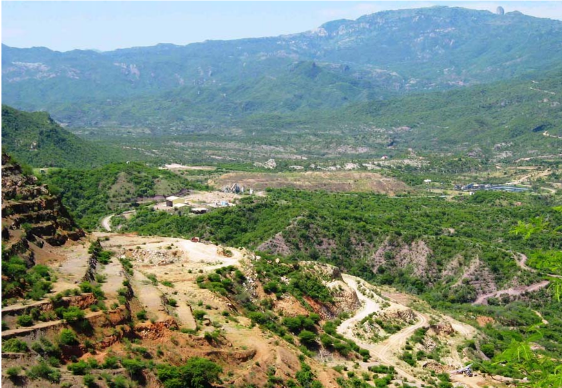
Fig. 4, Morris Mine Pit and Installations
