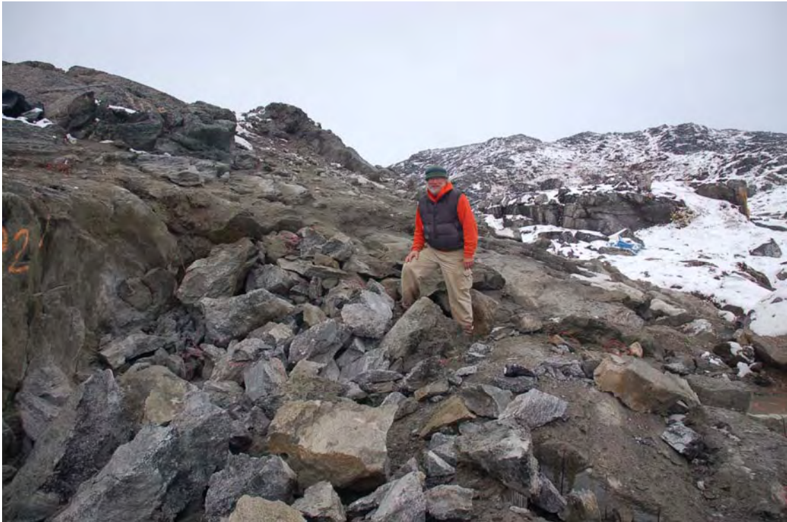
Illustration 19. Low yield blasting of 2nd 2007 bulk sample at Aappaluttoq – large blocks necessitate mechanical rock breaker in process plant to achieve maximum crusher feed size of 300mm to 400mm.
