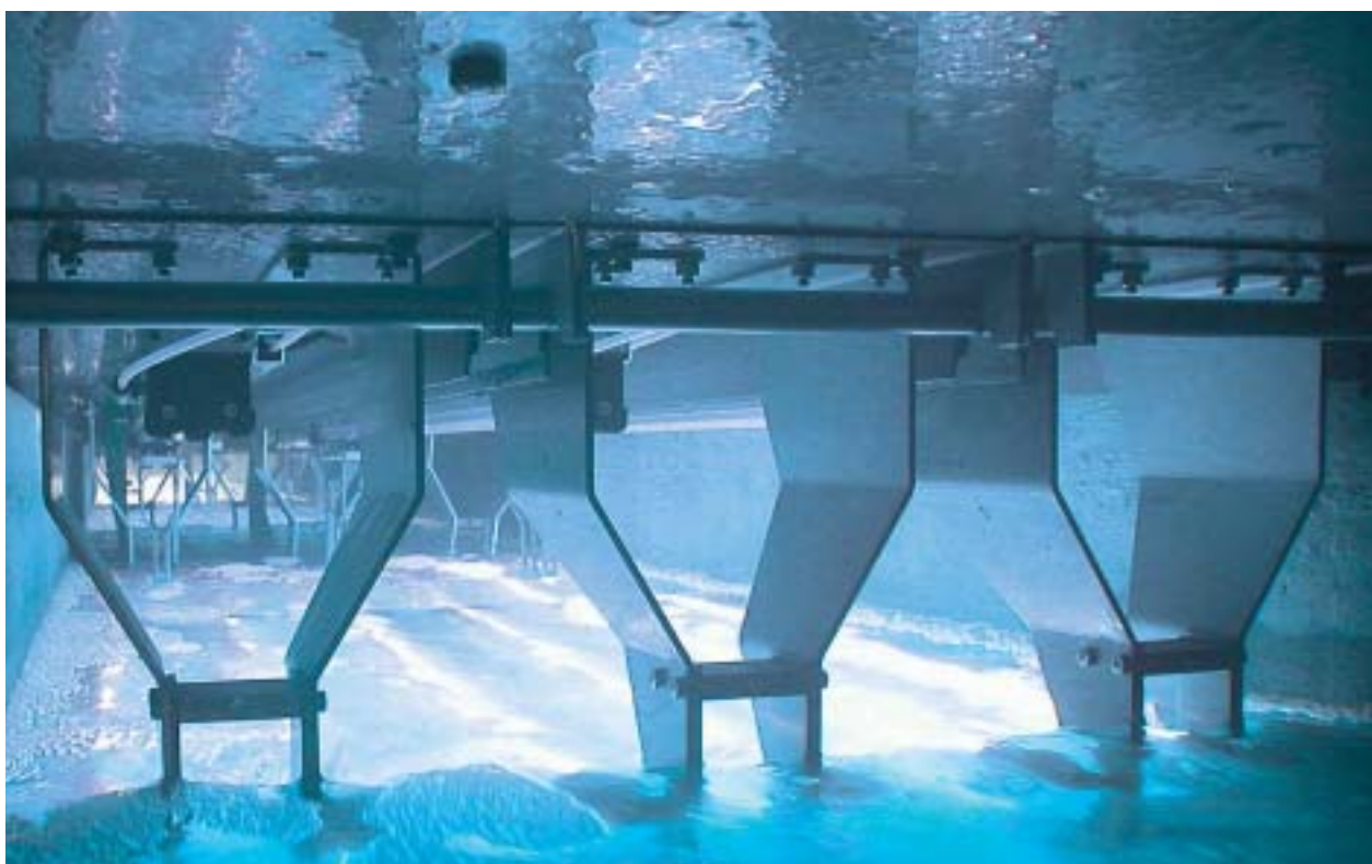
WEDECO UV system TAK 55 disinfecting waste water
